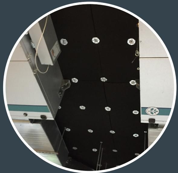
Pyrosorb is specified as a high performance acoustic barrier between walls and floors as pictured here – 25mm self-adhesive backed sheets adhered and fixed to concrete soffits between floors
